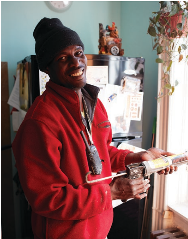
Preparing to caulk around a window
