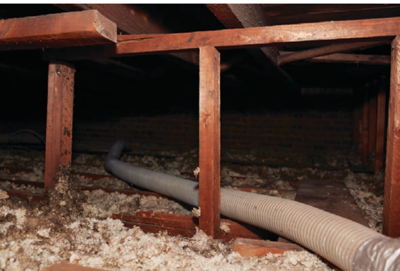
Adding cellulose insulation to poorly insulated attic cavity
