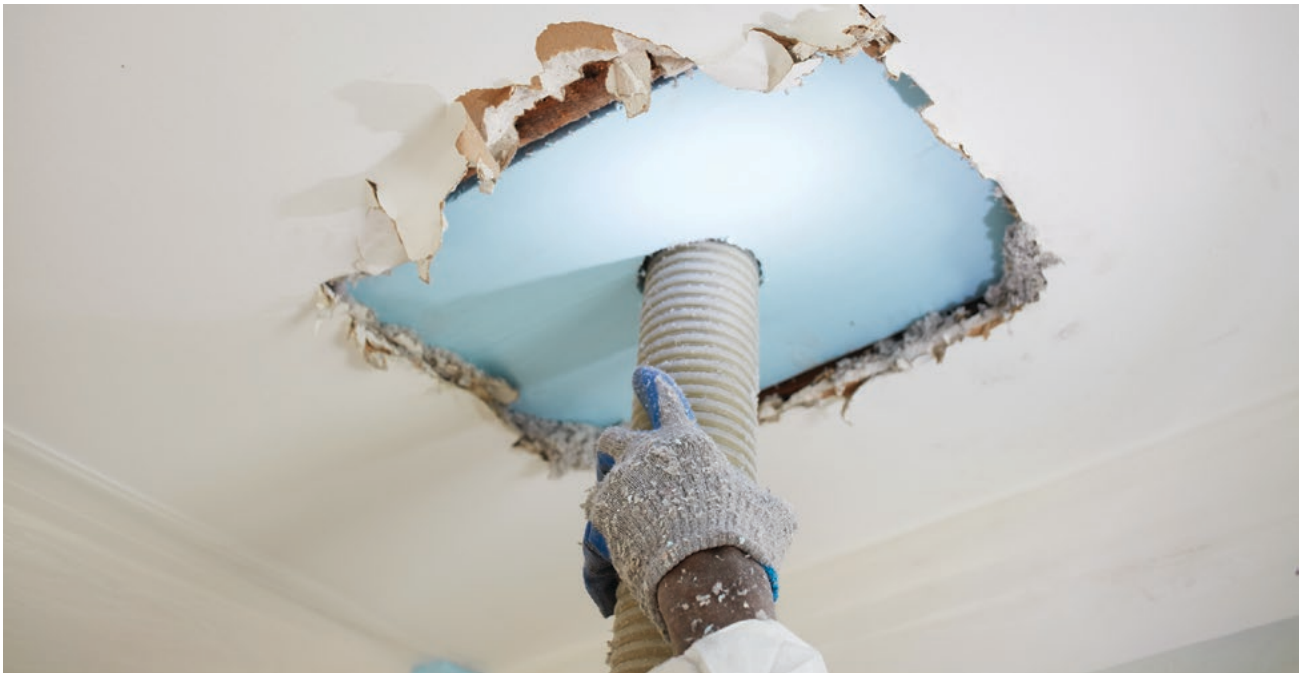
Blowing cellulose insulation into an attic cavity.
