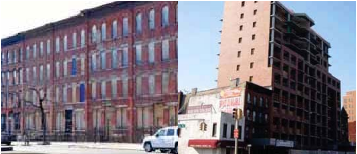
The subject buildings in 2007 (left) and luxury housing development 2010 (right)
