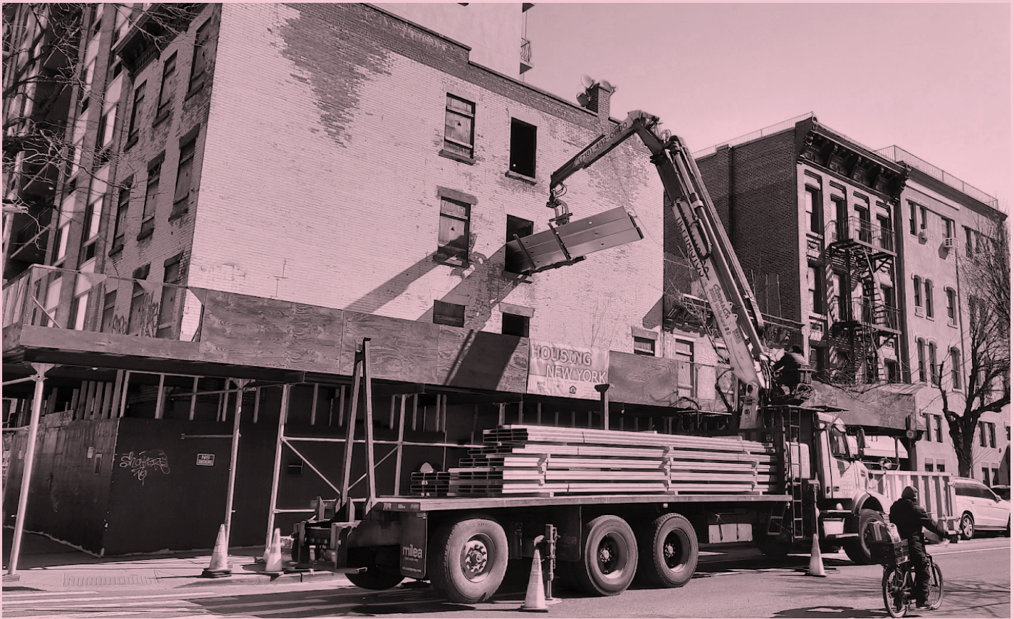
Rehabilitation of apartment buildings on the East Harlem-El Barrio CLT, 2021
