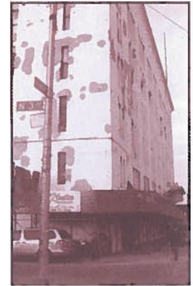
184 Kent Street in Williamsburg is a six-story industrial building that has been converted to residential use.
